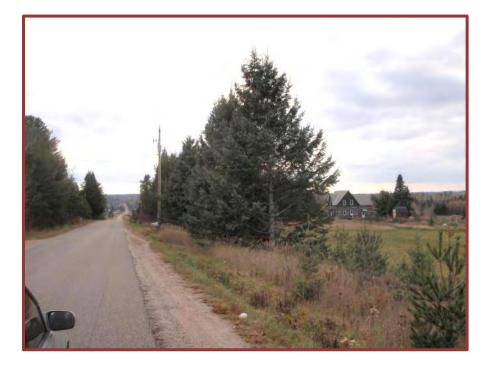
Image 112: Looking West Along Highway 17 Towards Rutherglen (note: steep and ditched gravelled shoulders)
