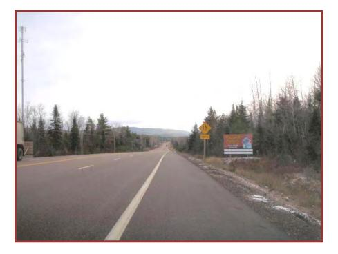
Image 79: Looking East Down Highway 17 (note: deep ditches, sloped, gravelled and paved shoulders)
